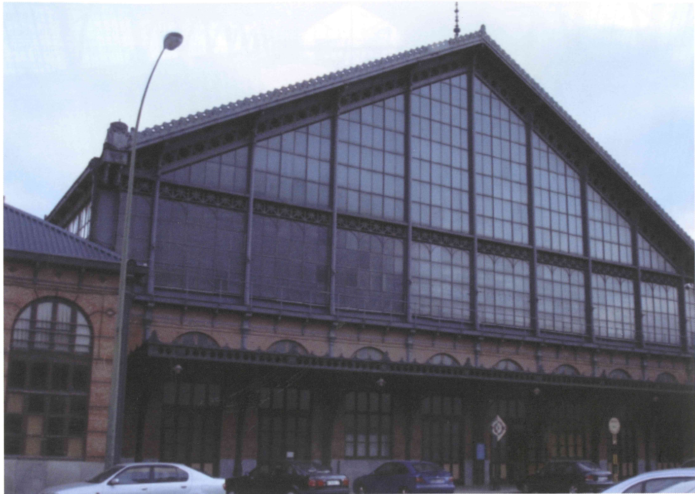
The old Delicias station in Madrid, a magnificent example of the “iron architecture” of the nineteenth century and site of the Madrid Railway Museum
