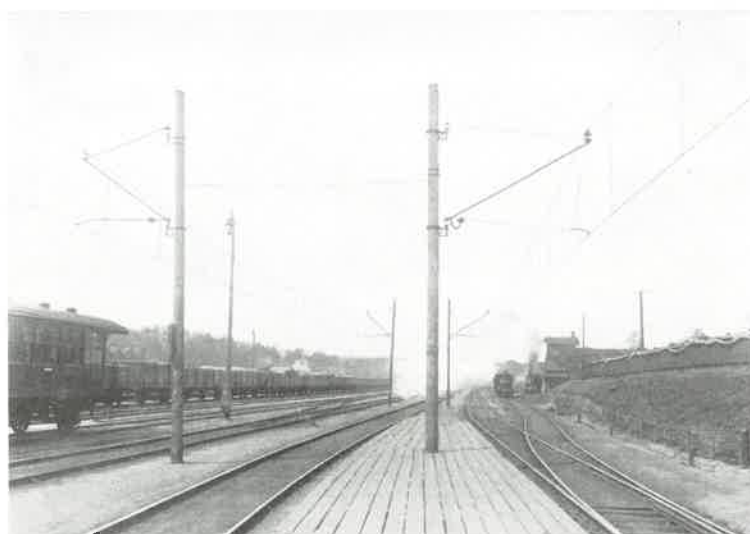
Fig. 1. Overhead line on the experimental railway Stockholm—Tomtebodavärtan—Järva. Indirect support, double insulation.
