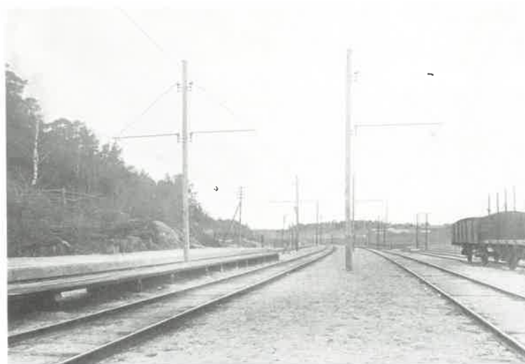
Fig. 2. Overhead line on experimental track. Direct support, single insulation, flexible system.
