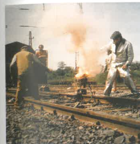
Figure 21. Railways superstructure modernisation (rail-welding)
