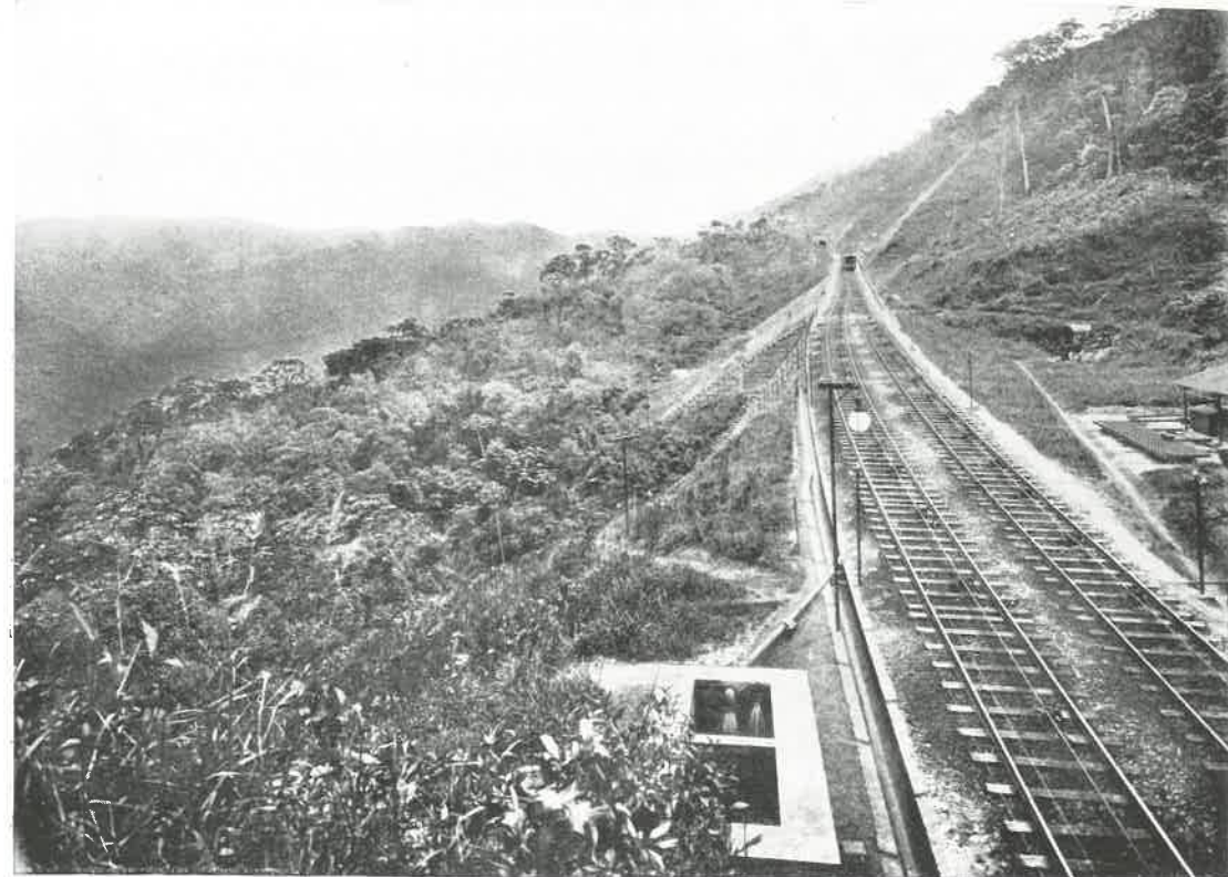
PASSING PLACE ON THE INCLINE, SHOWING UP AND DOWN TRACKS AND CABLES.
